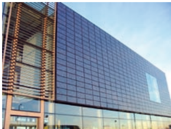
PV cladding is part of the new Manchester College of Arts and Technology (MANCAT) building, UK
