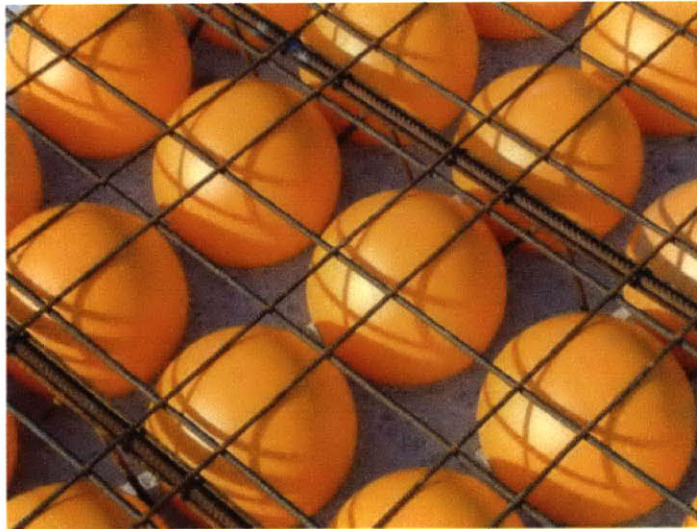
Figure 3-1: Components of a BubbleDeck (Stubbs)
