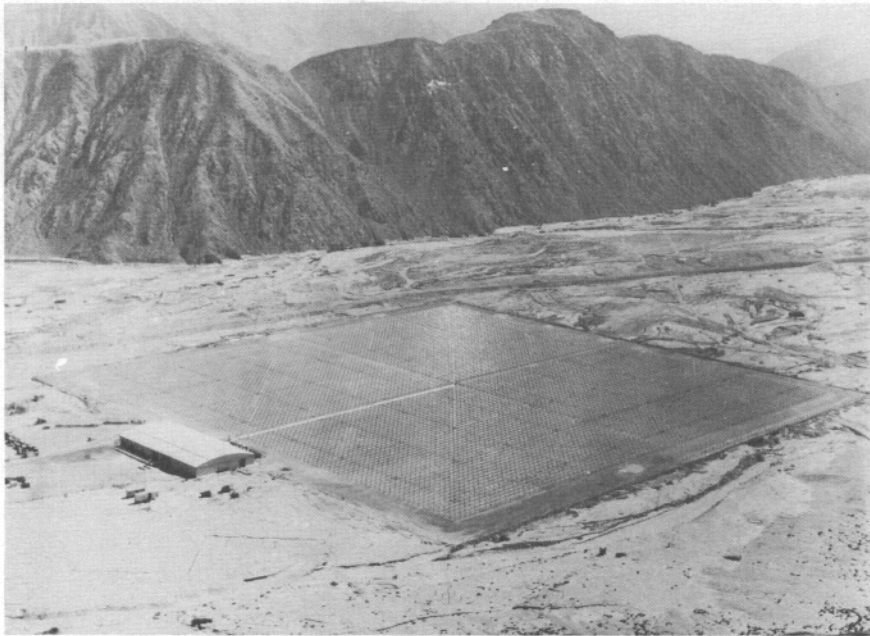
Fig. 7. A view of the Jicamarca radar facility in Peru. The antenna is a square array of dipoles, 300 meters along a side. The building houses the transmitter, receivers, and data processing equipment. (Courtesy of ESSA Research Laboratories, Boulder, Colo.)
